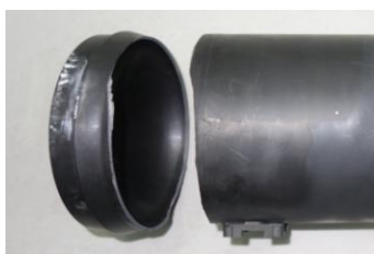
Figure 1. Transverse breakage shell
